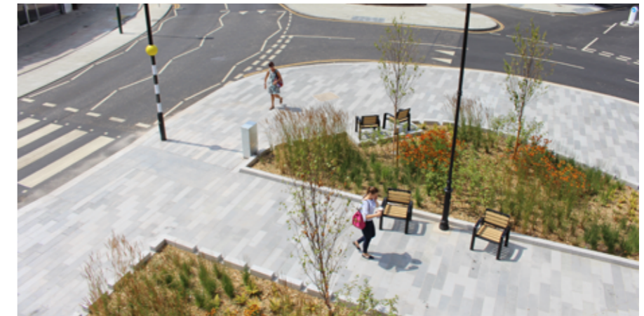
Sensory Rain Garden in Gidea Park, Havering designed in space reclaimed from road space at a redesigned junction provides a communal green node and a functional SuDS feature.
