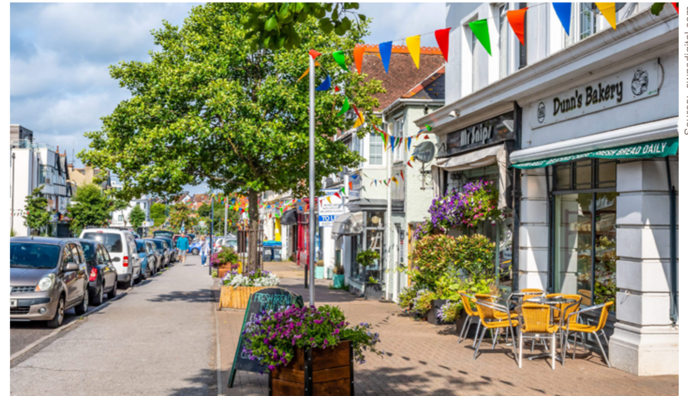
Example of a Linear Place in Tankerton High Street, Whitstable, Kent with shops activating the street, high quality public realm and landscape treatments.
