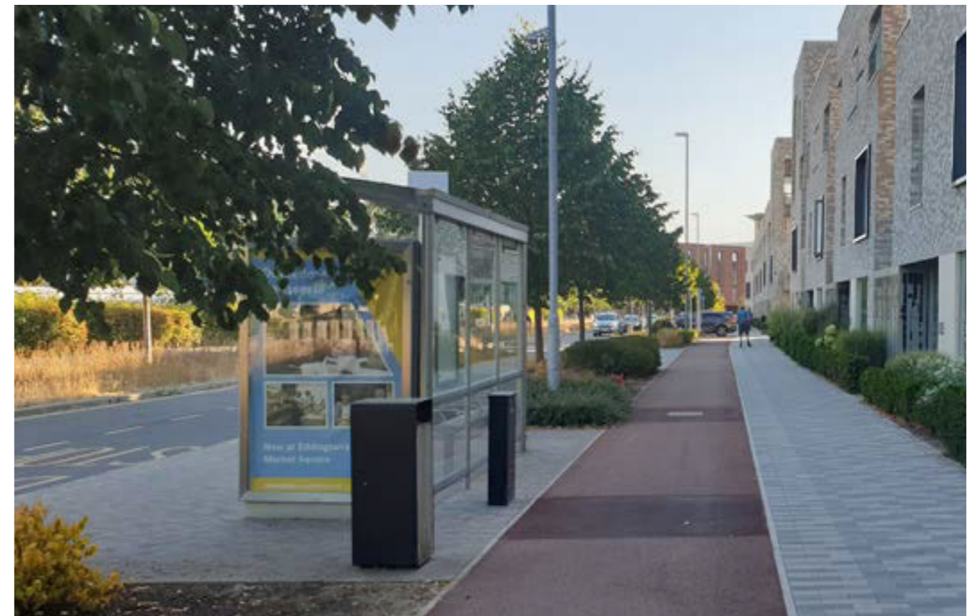
Example of a Mixed-Use Street with a bus stop, a wide cycle lane and well designed footway along residential frontages.
