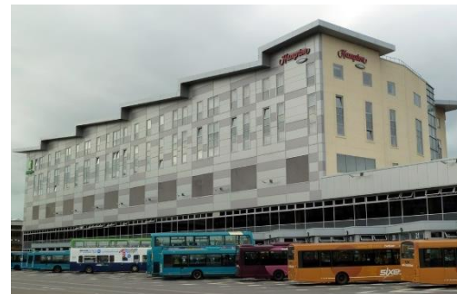
Derby Bus Station; Derby, UK
