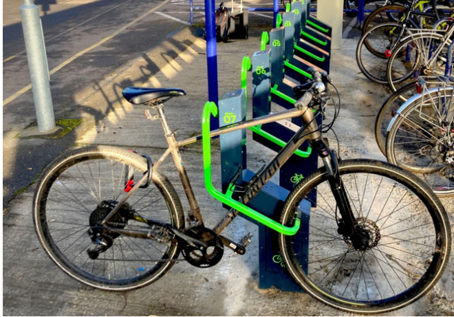
Figure 4-6: Electric bicycle parking and charging 27
